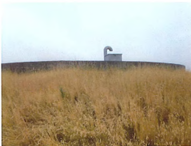
Photograph 11: Partially Buried 125K Concrete Storage Tank
