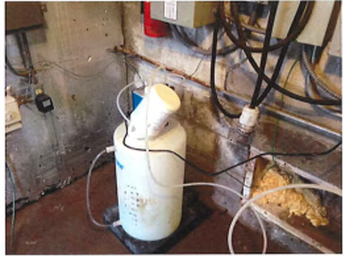
Photograph 4: Chlorinator Tank
