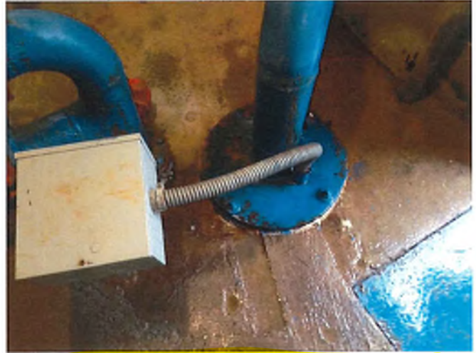
Photograph 2: Well 1 Casing is Flush with the Ground Surface
